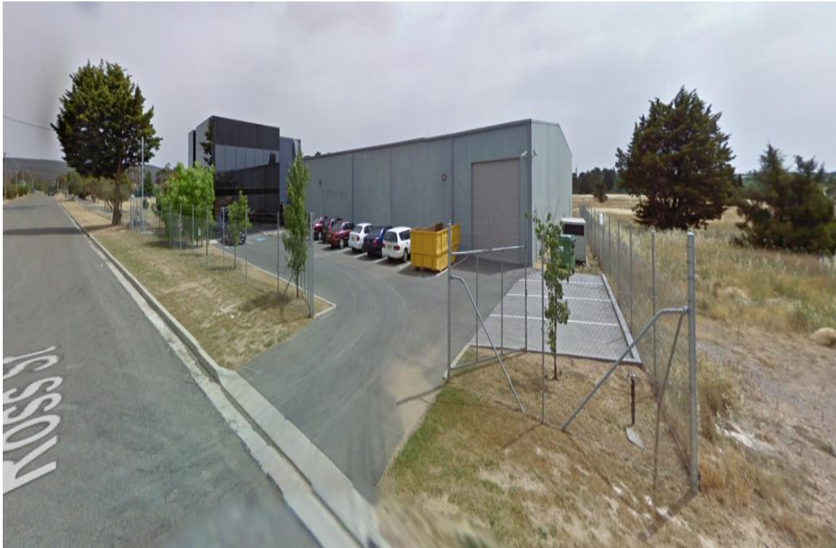
View of the existing building to the South of the property.
